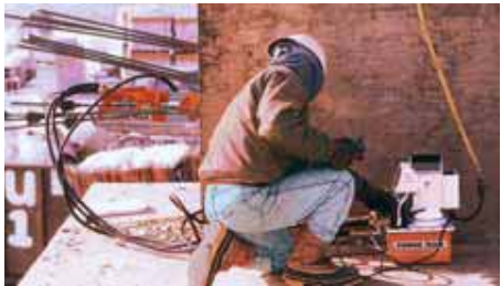
The PE60 used for pre-stressing.
